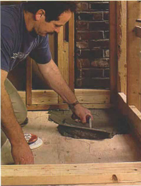
Thinset begins the shower pan. After the subfloor has been swept clean, a layer of latex-modified thinset is applied to bond the layer of mud that follows.
