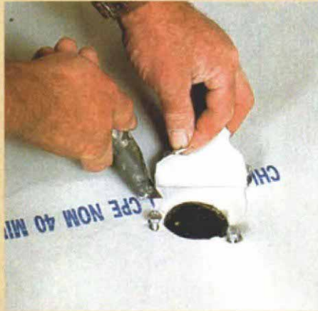
Cut in a circle between the bolts.
