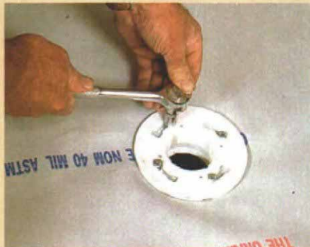
Tighten the bolts.
